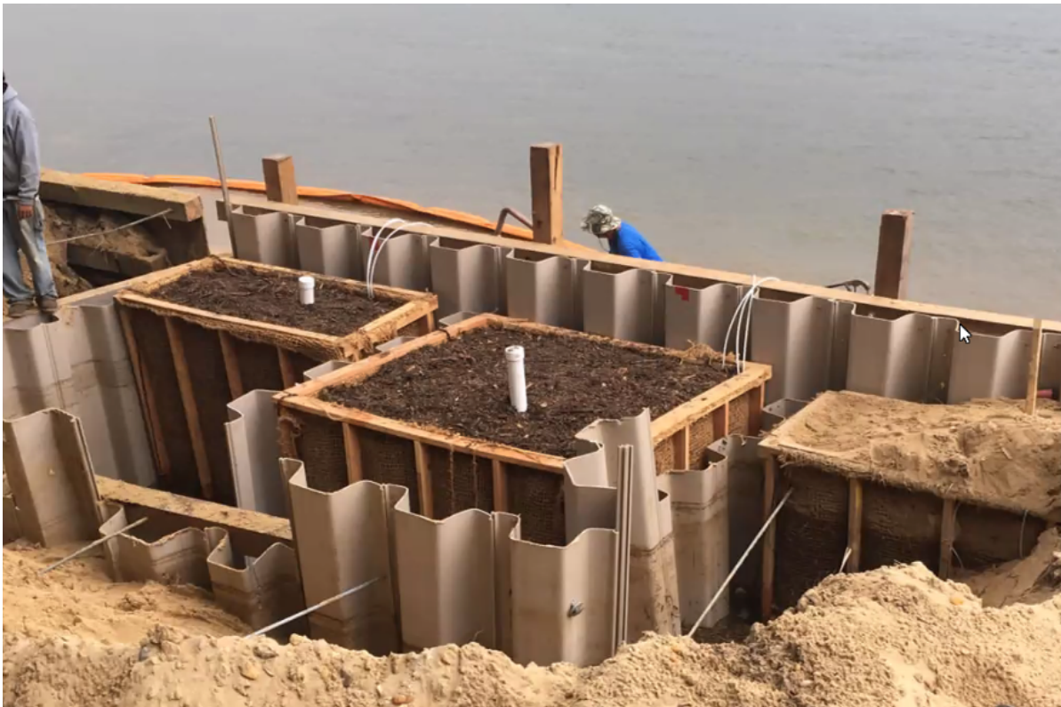
Figure 15 - Permeable Reactive Barrier (bulkhead under construction)
