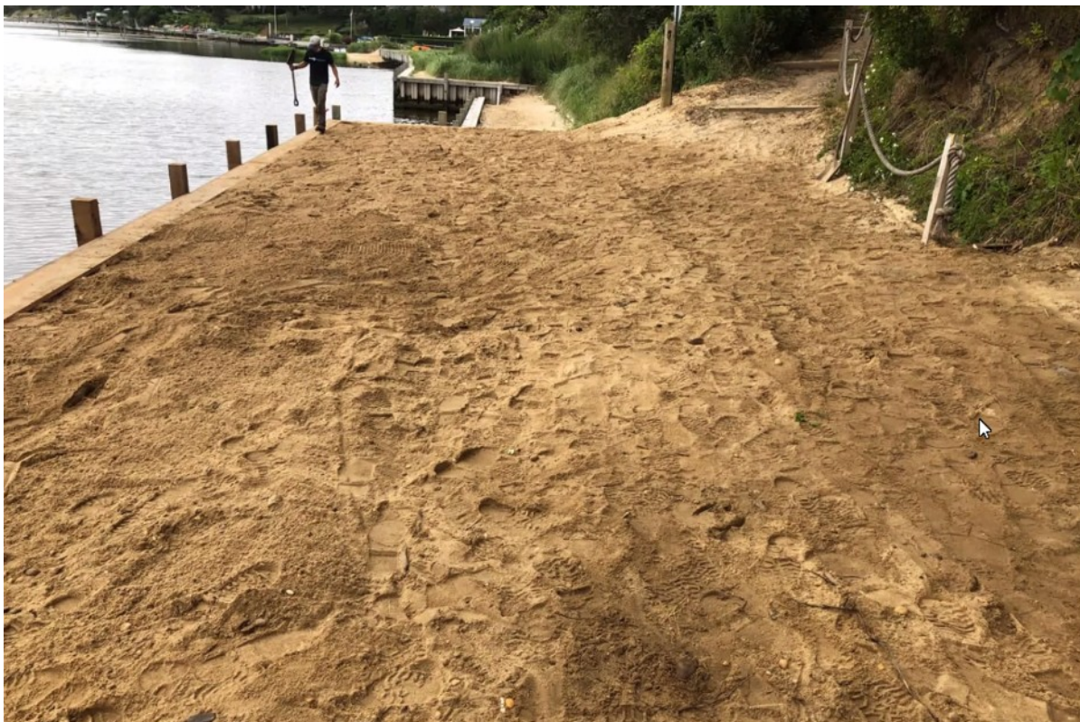
Figure 16 - Completed Bulkhead PRB
