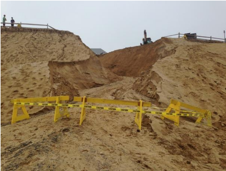
Figure 2.5 | Cahoon Hollow parking lot and dune erosion.
