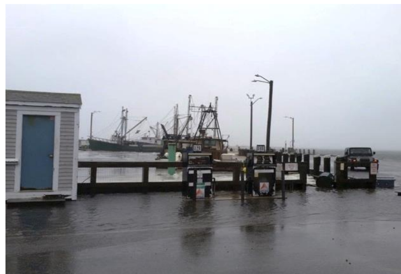
Figure 2.13 | Storm surge at Wellfleet Harbor, January 2018 Nor'easter
