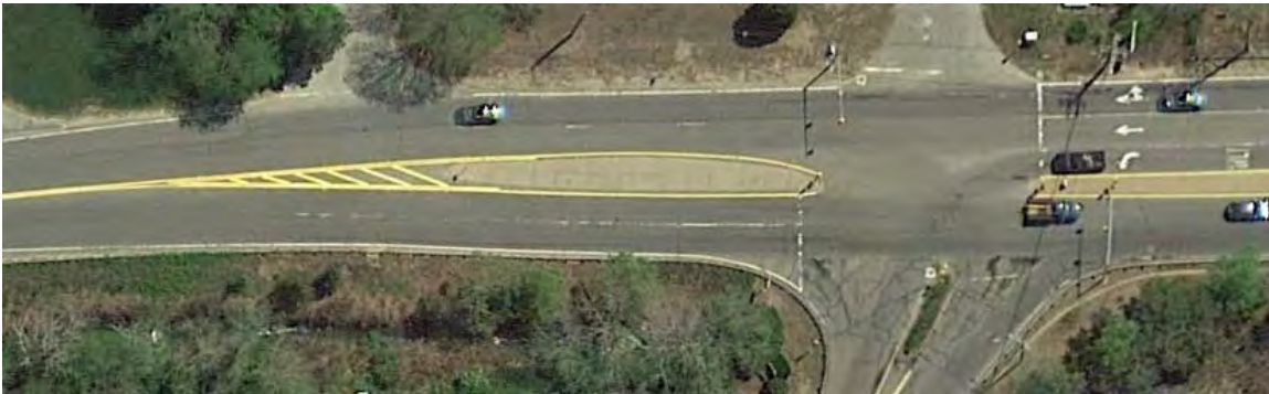
Figure 13 - Aerial view of Route 6 north of Main Street (north to left)
