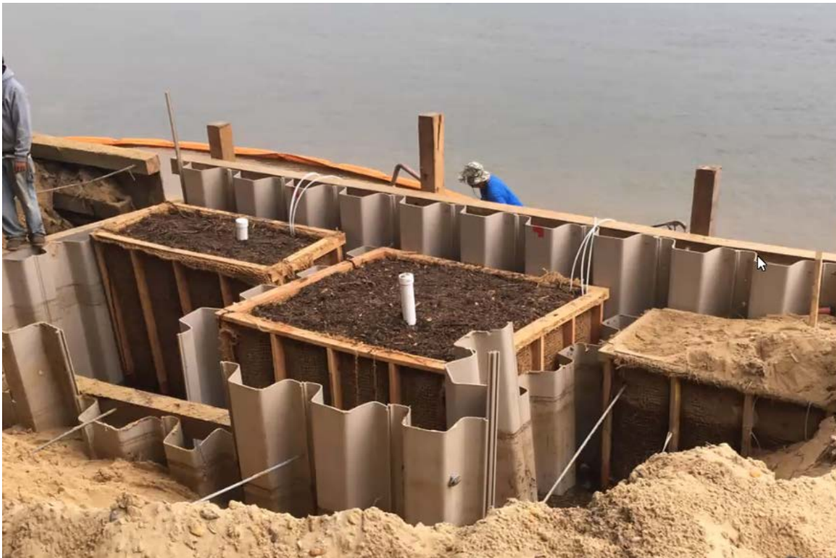
Figure 15 - Permeable Reactive Barrier (bulkhead under construction)
