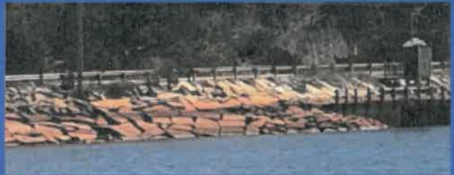
Existing Stone Revetment
