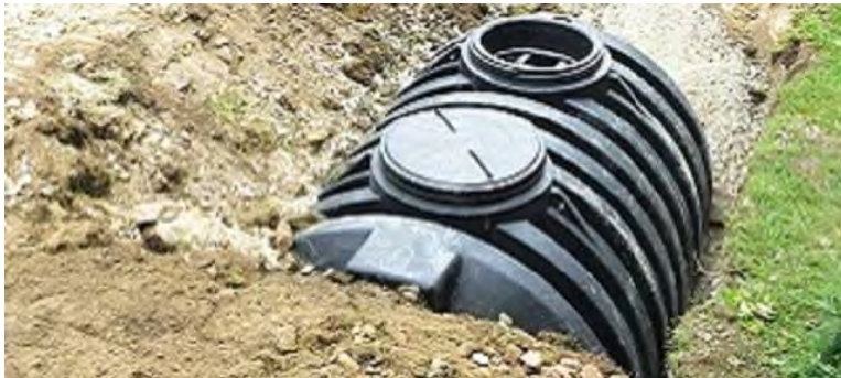
Figure 38. Septic system (US Environmental Protection Agency).
