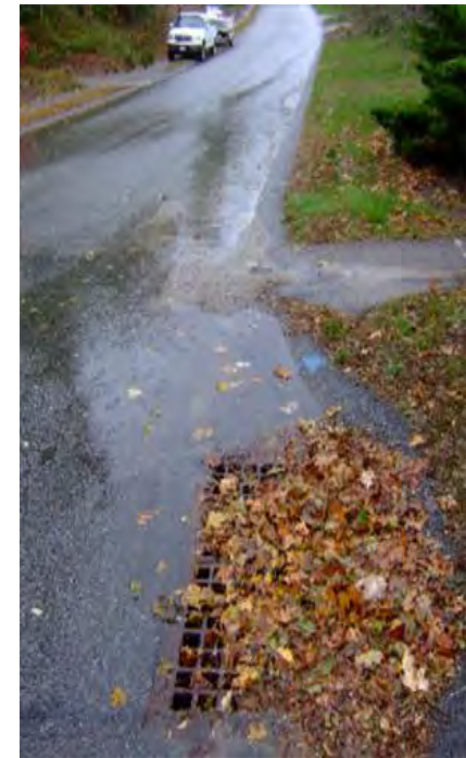
Figure 26. Stormwater runoff carries debris down to the storm drain (Association to Preserve Cape Cod).
