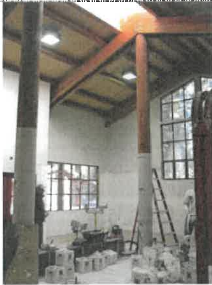
Building construction and interior finish
