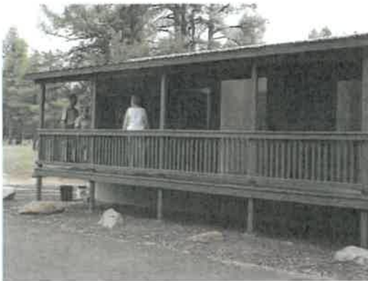
New shower building
