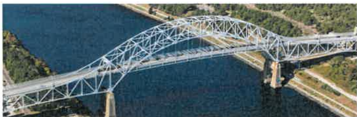
Learn more about the new Canal Bridges Task Force: cecom.link/bridges-task-force
