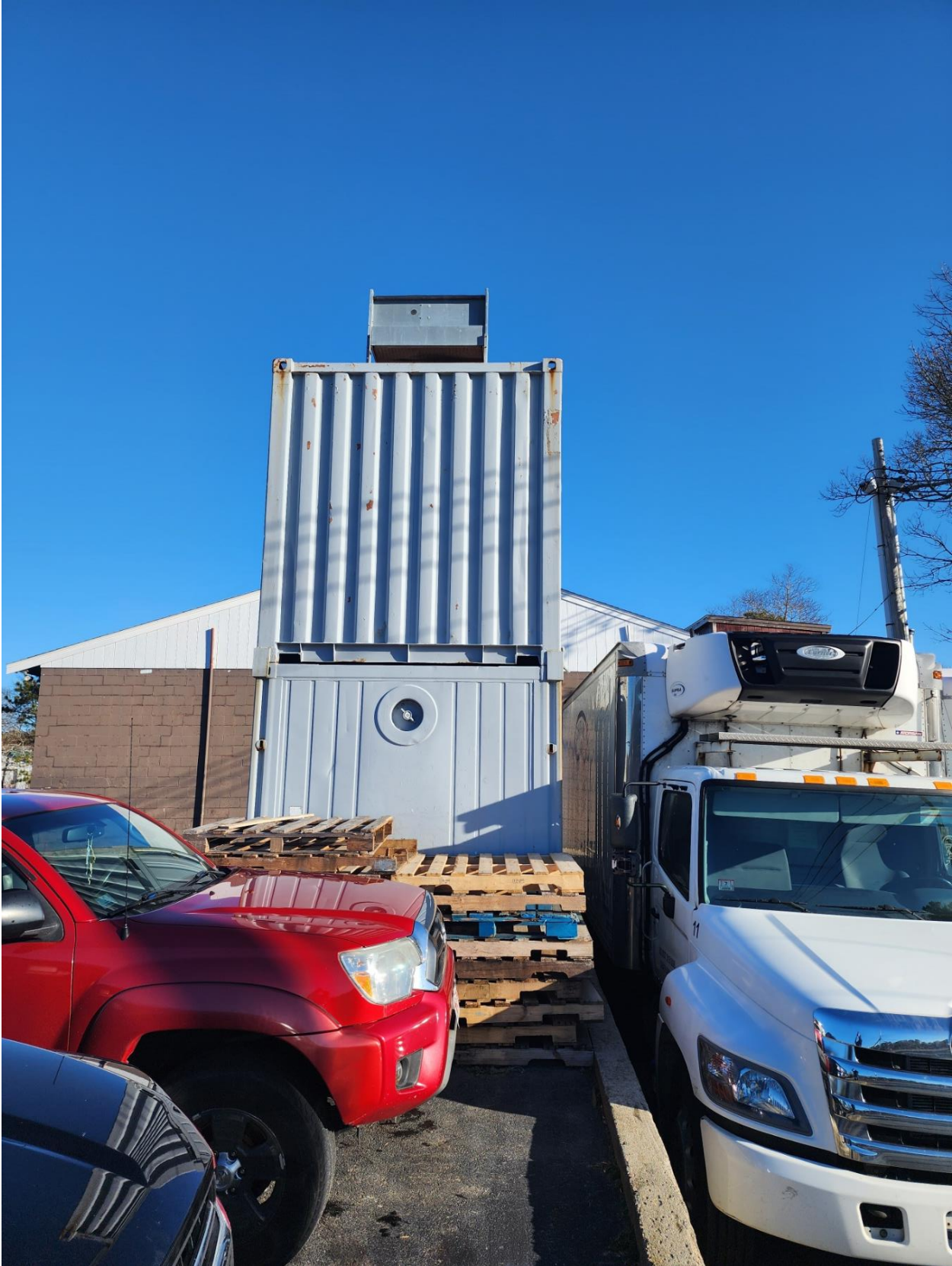
Figure 3 Typical installation - double stacked shipping containers
