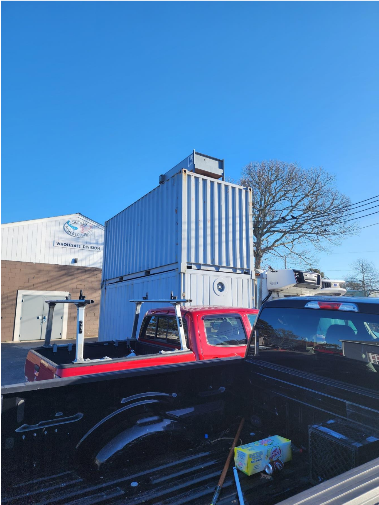
Figure 4 Condensing Unit is mounted on top. Ice Maker is installed in upper container. Lower container is for ice storage
