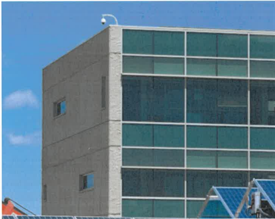
Mass wall (gray, left), spandrel (light blue, between floors), and vision glazing (darker blue).
