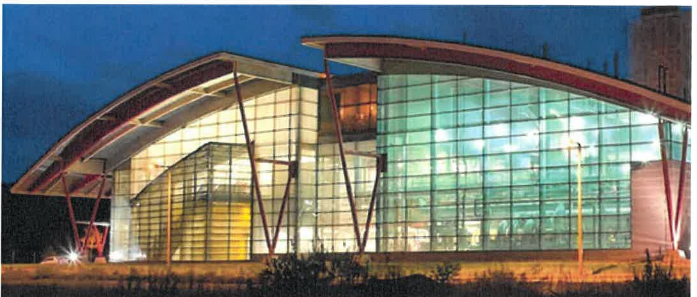
The University of Massachusetts Amherst Central Heating Plant, pictured above, provides 70% of the campus' electricity and 100% of its steam needs from natural gas. In the future, district heat systems such as this could operate using the dual-fuel approach that leverages electric boilers when renewable energy is abundant and low-carbon gas at other times. Photo credit: UMass Amherst
