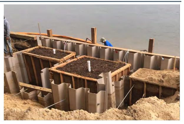
Figure 15 - Permeable Reactive Barrier (bulkhead under construction)
