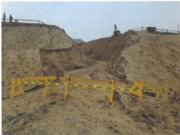
Figure 2.5 | Cahoon Hollow parking lot and dune erosion.
