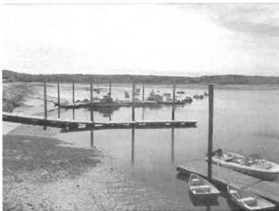
North Anchorage and Boat Ramp
