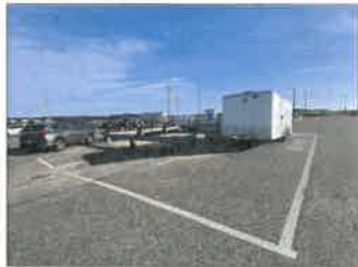
1. OVERALL VIEW OF FUEL STORAGE TANK AREA
