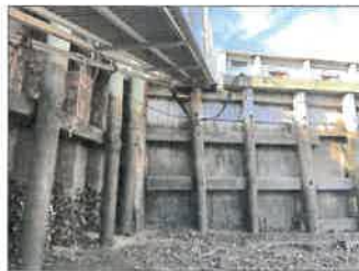
7. EXISTING FUEL LINES UNDER GANGWAY
