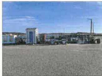
3. OVERALL VIEW OF EXISTING DISPENSER STATION
