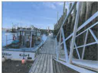
9. OVERALL VIEW OF FUEL FLOATING DOCK
