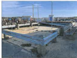
2. OVERALL VIEW OF FUEL STORAGE TANK AREA
