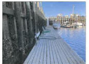
12. OVERALL VIEW OF FUEL FLOATING DOCK LOOKING SOUTH
