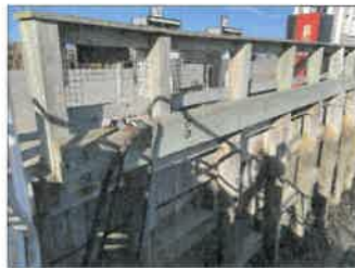
6. FUEL LINES AT BULKHEAD ADJACENT TO DISPENSERS
