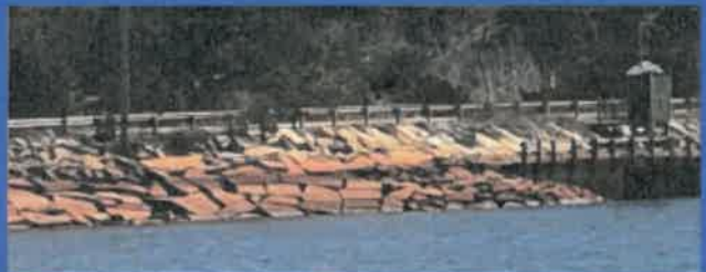
Existing Stone Revetment
