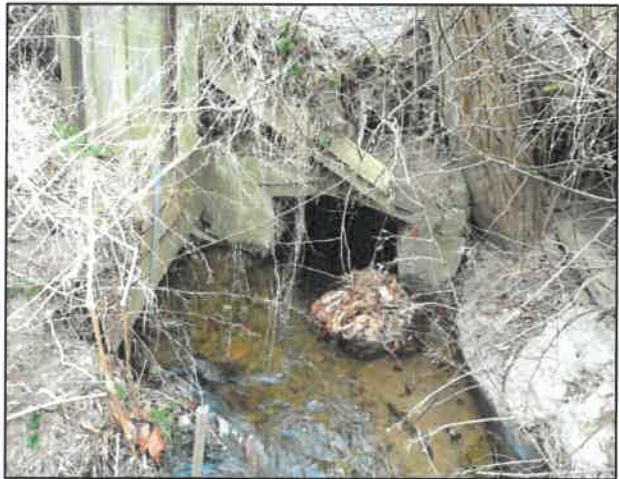
Outlet and Downstream Headwall of Old Kings Highway Culvert ( J. Portnoy 2019 )
