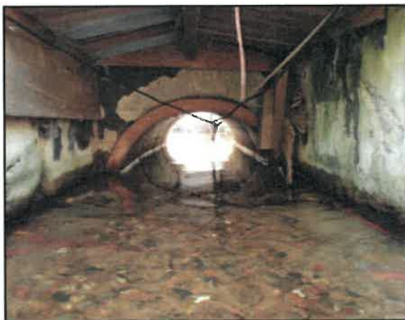
Inside of Old Kings Highway Culvert from downstream ( Stantec, 2014 )
