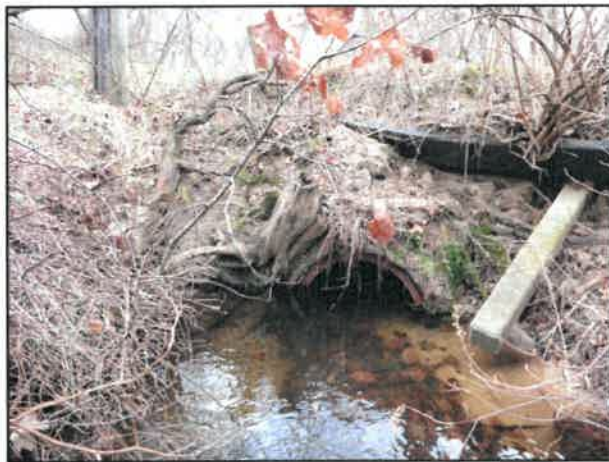
Inlet to Old Kings Highway Culvert (J. Portnoy 2019)
