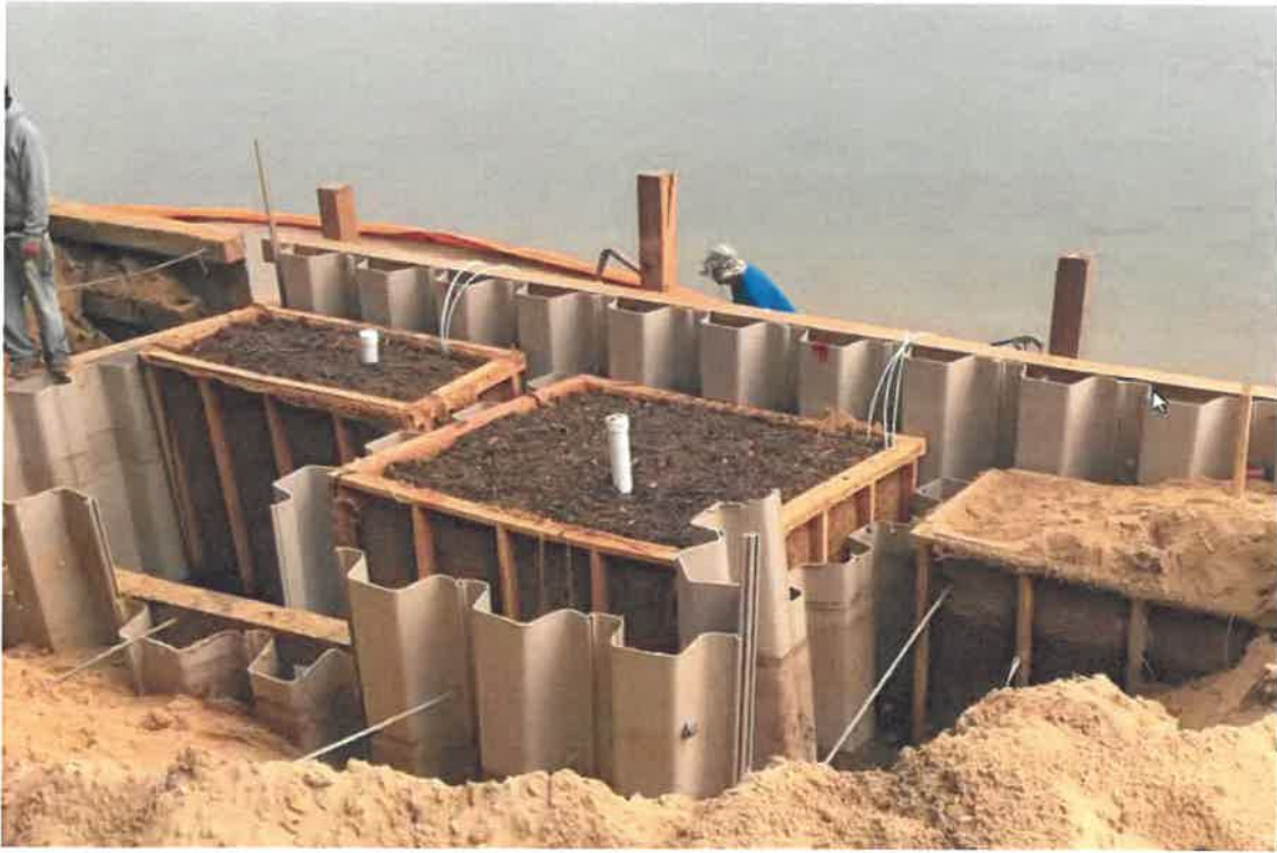
Figure 15 - Permeable Reactive Barrier (bulkhead under construction)
