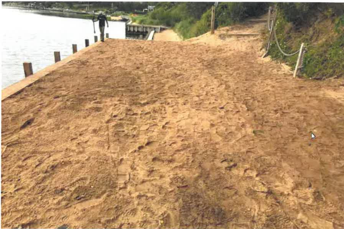
Figure 16 - Completed Bulkhead PRB
