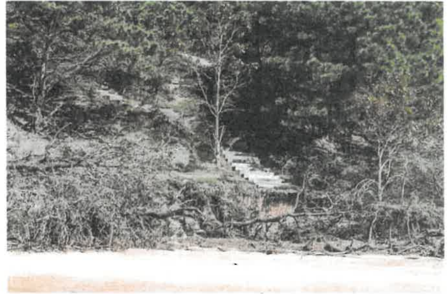
Photo showing the Prager beach access steps on 10/11/21
