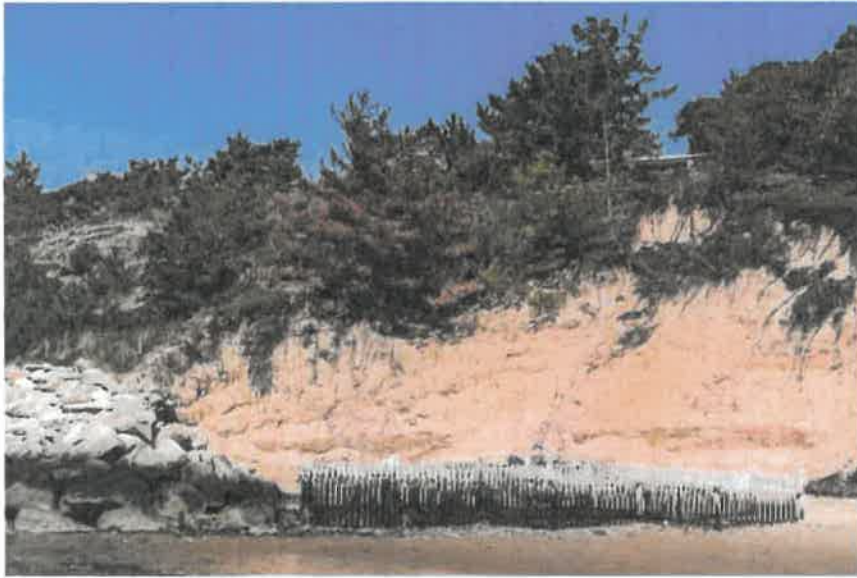
Photo showing existing conditions on 10/11/21
