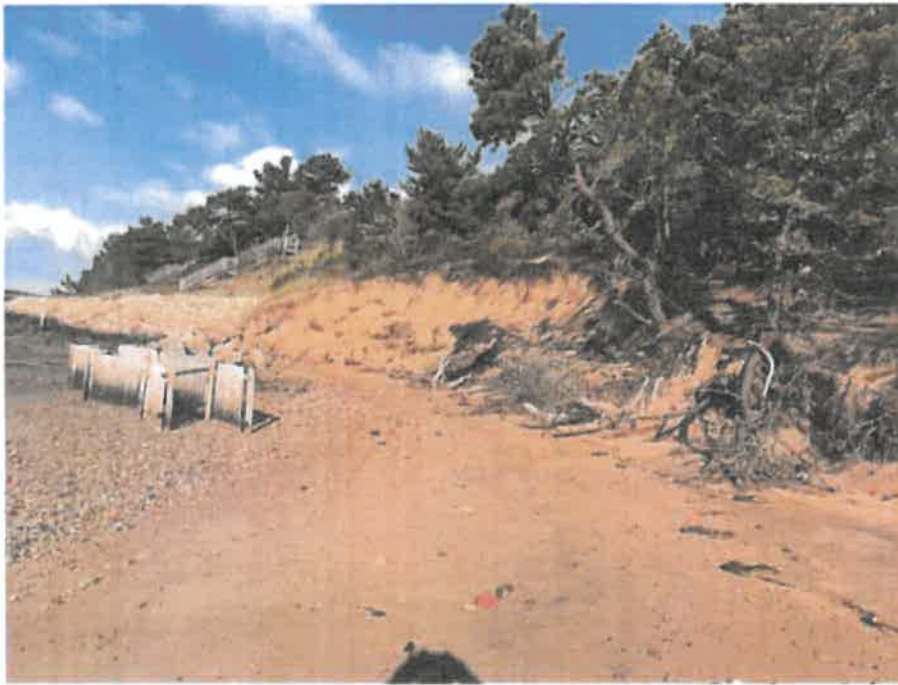
Photo showing existing conditions on 10/25/18
