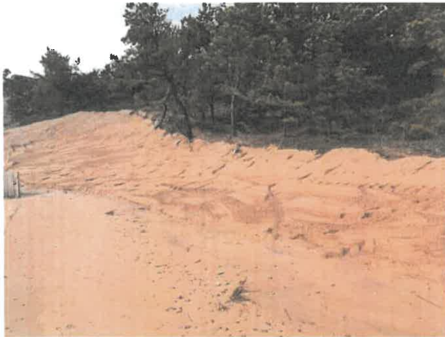
post nourishment condition on 3/12/18 (800 cubic yards)
