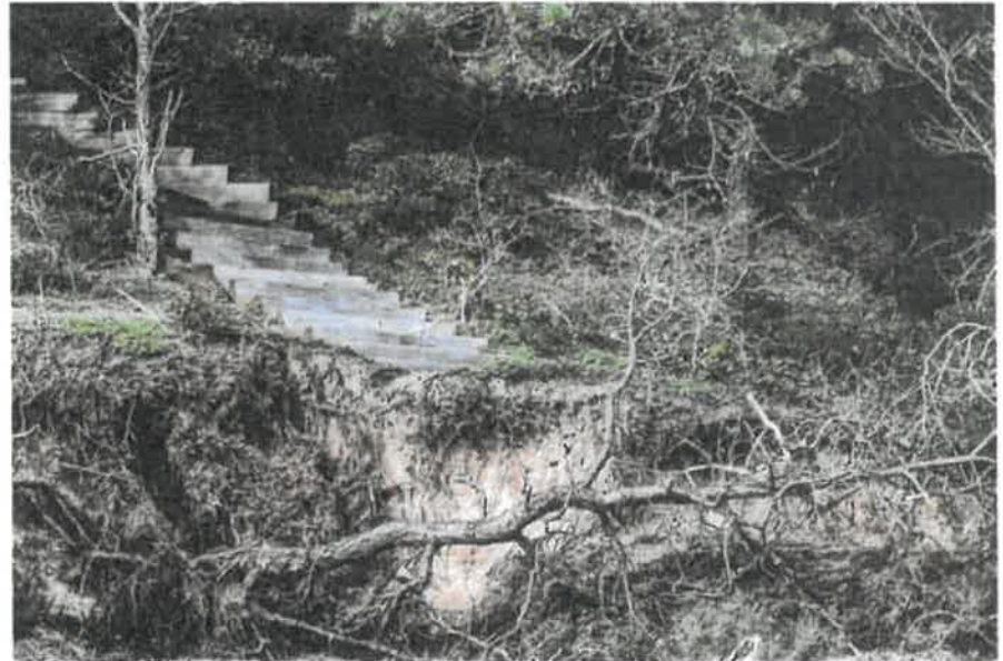
Photo showing the Prager beach access steps on 9/2/21
