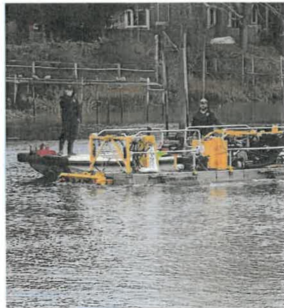
Pocasset River Dredge, Bourne, MA
