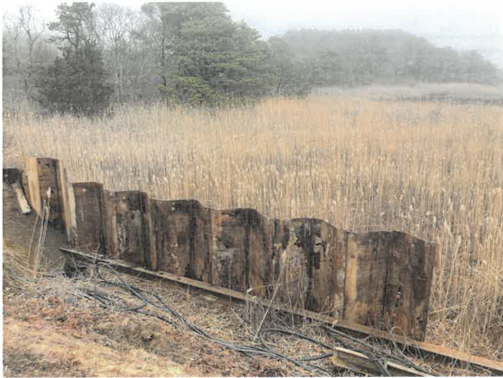
Figure 1. – Showing steel sheeting installed as MIG works from the Duck Harbor Road staging area towards the river.
