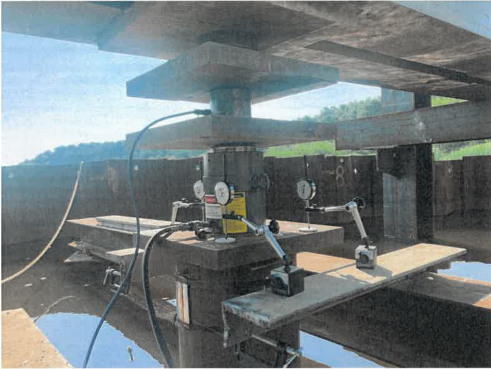
Figure 5. – View showing permanent test pile load testing setup.
