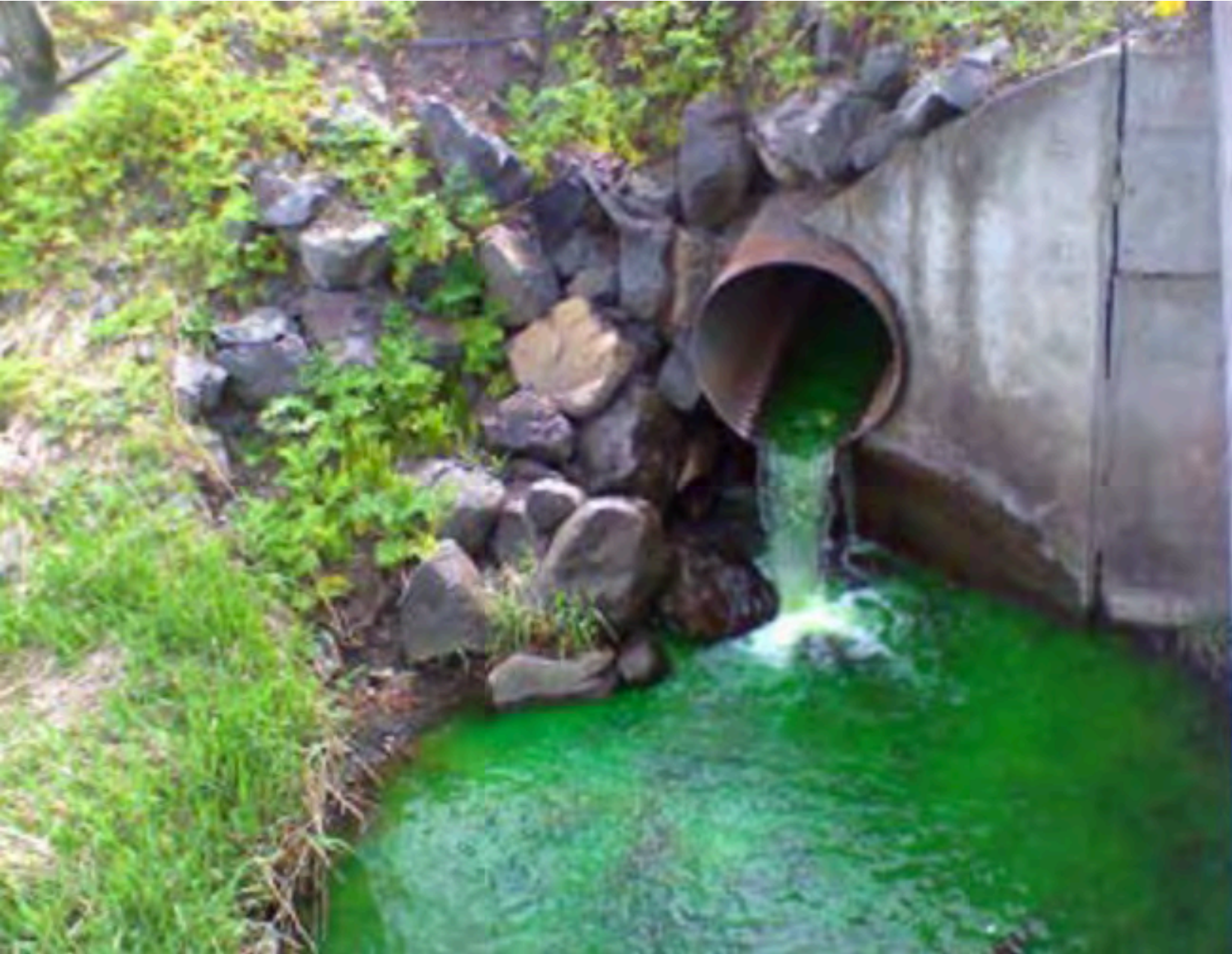
Stormwater Remediation Projects
