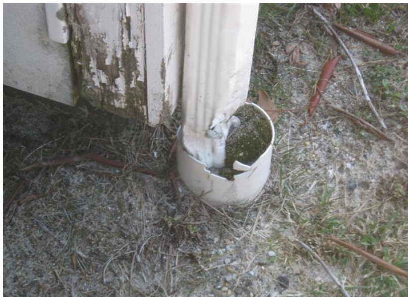
Voids in the rotting wood trim boards allows water to seep behind siding and be absorbed by sheathing
