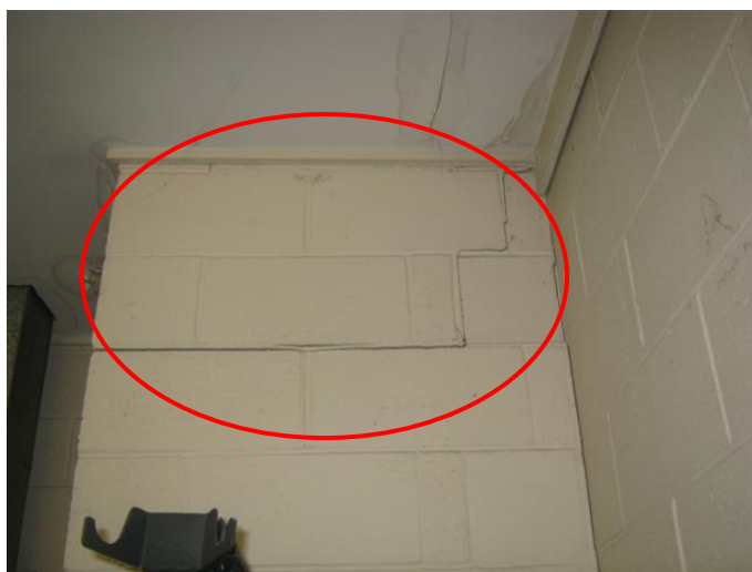
Horizontal and step crack at chimney wall
