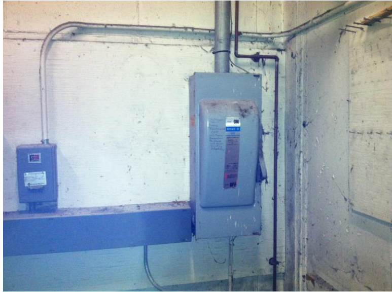
Code violation of water line directly over main disconnect switch.
