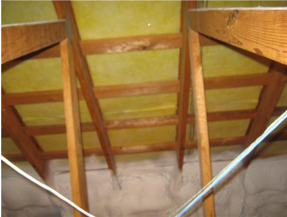
Wood blocking at top chord of main trusses for support of piggyback trusses above
