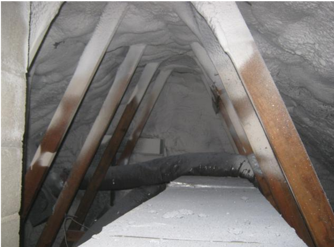
Close up of sprayed on insulation which conceals underside of roof deck sheathing
