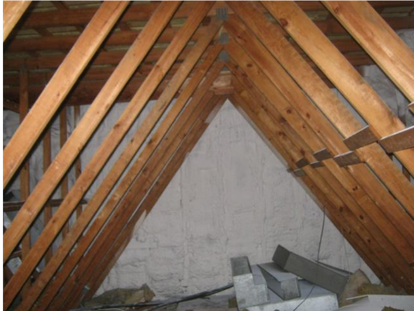
Typical wood roof truss
