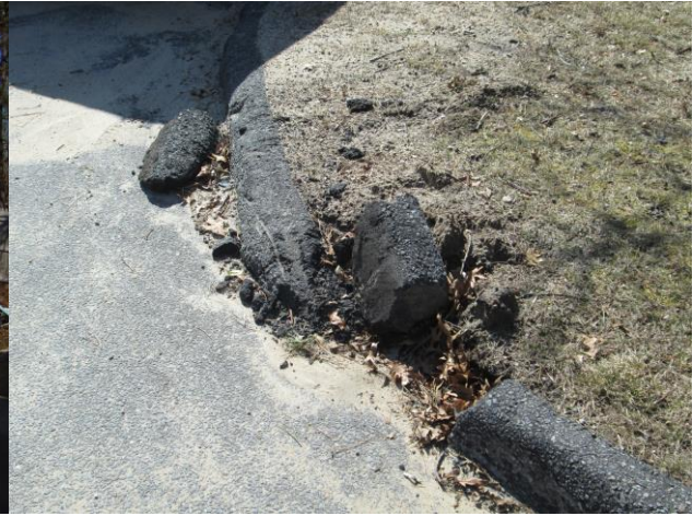
Damaged asphalt curb
