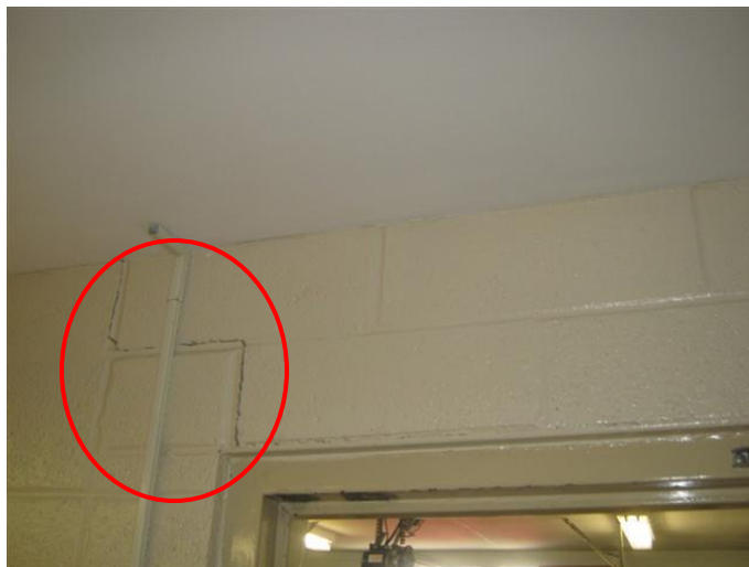
Cracks in concrete block wall adjacent to door opening
