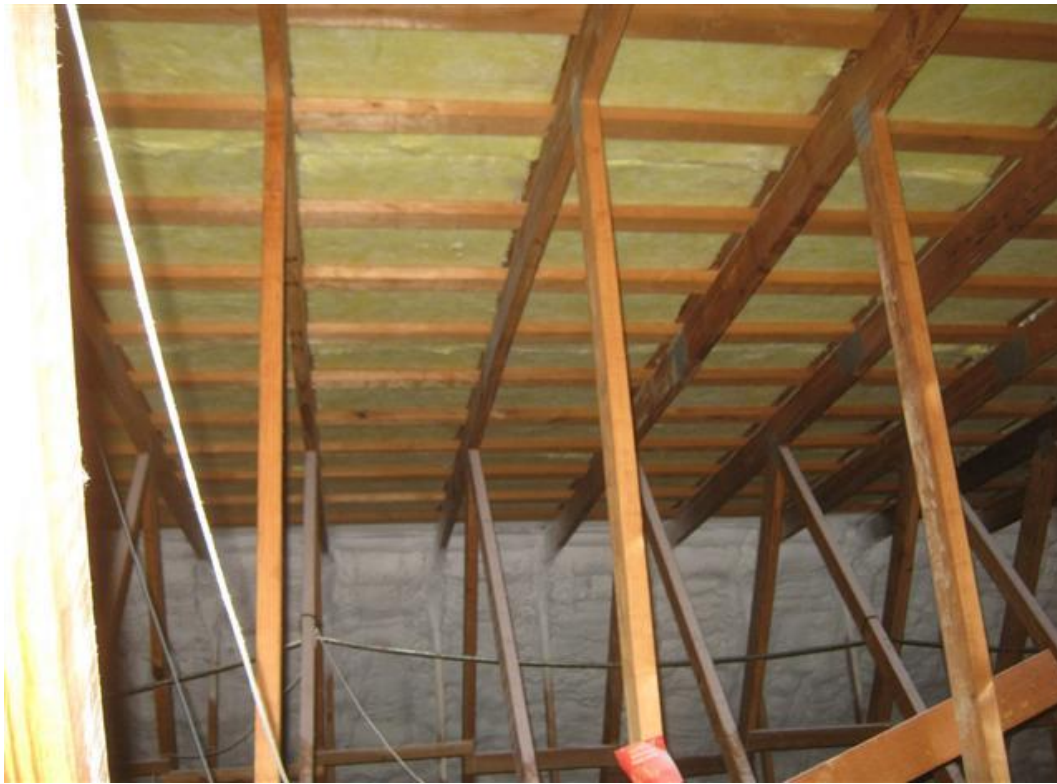
Insulation board on top chord and sprayed on insulation in the background
