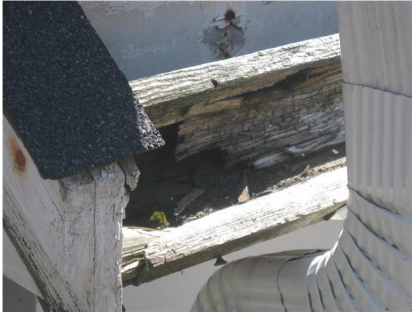
Deteriorated wood gutter allows infiltration of water into building
