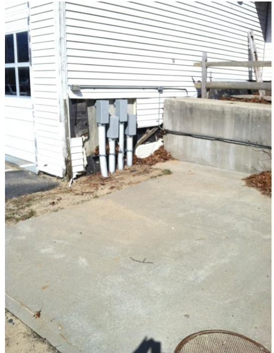
Underground conduits to fire department across street.
