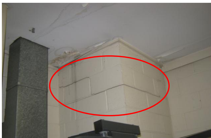
Horizontal and step cracks in concrete block walls of chimney
